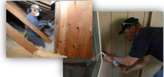
Air Leakage Control Installer (RBE-WHALCI)
